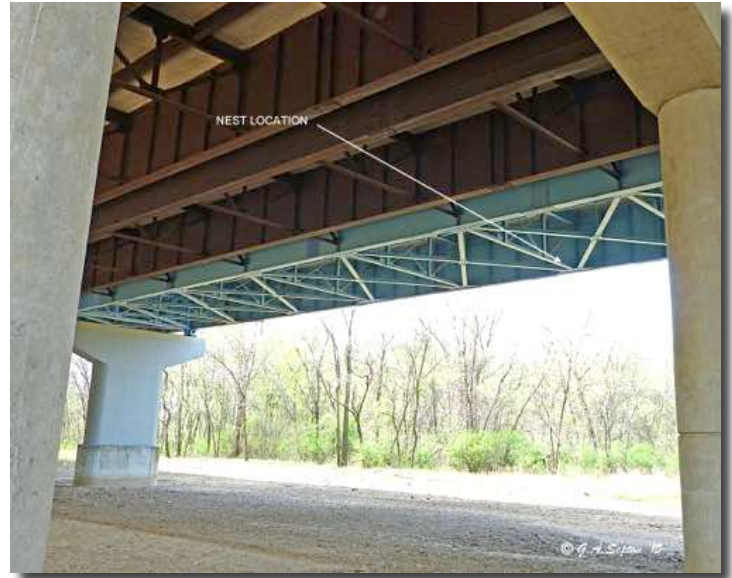
Above: The nest site location under the bridge
