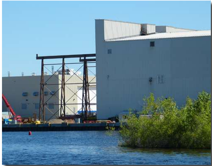
Above: The MMC site showing I-beams that support a crane hoist. The suspected nest site is atop a column beneath where the I-beam enters the building
