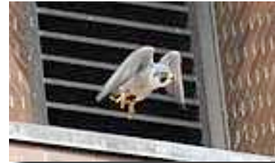
Above: The upper ventilation ducts at the Cofrin Library Below: An adult peregrine leaving the nest ledge
