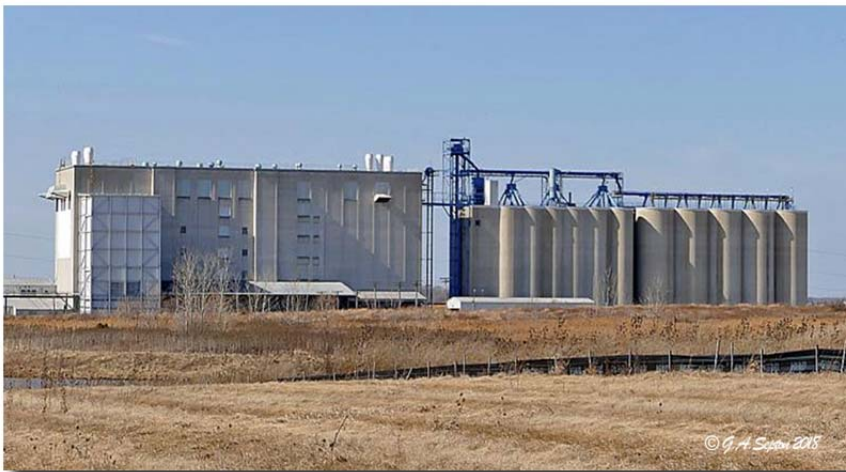
The Ardent Mills site with its tall elevator and silos should be an attractive site for peregrines. With a new nest box in place, we'll know more come spring.
